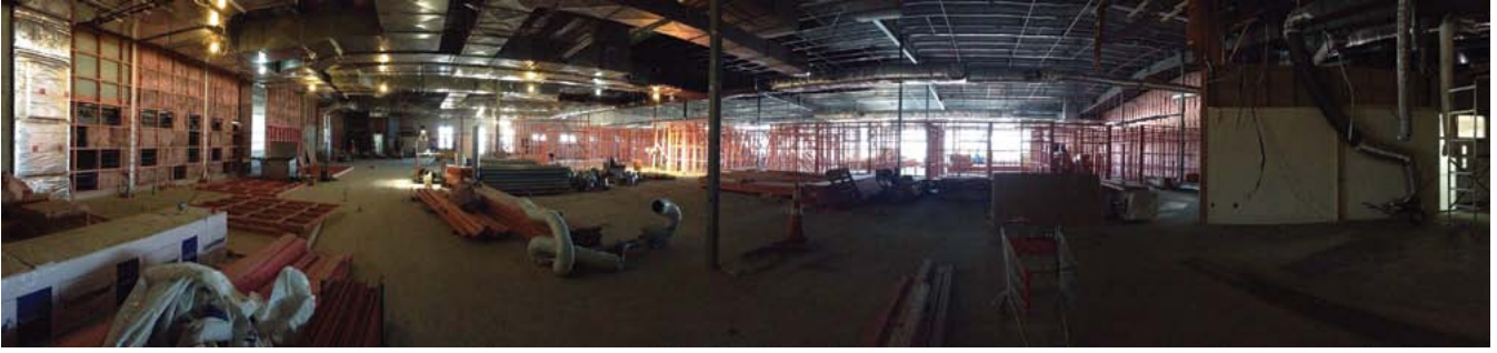
Construction is well under way.
